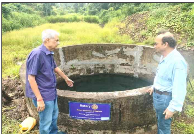
Water level of Farm Pond
