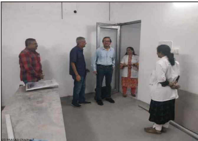
Modular OT work in progress
